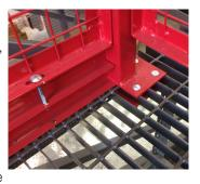
growth plates can be cut and notched in the field, as required.
